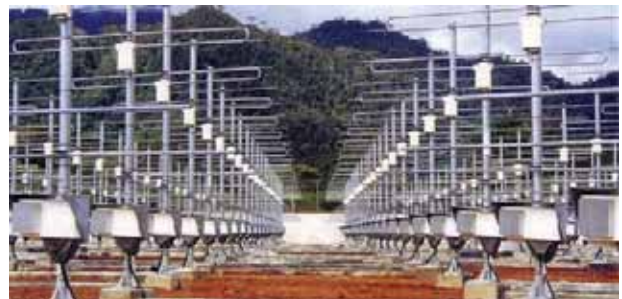
Figure 3. Three-element Yagi antennas are shown, each with a transmitter-receiver module (TR modules) mounted, near the ground, on the pole.
