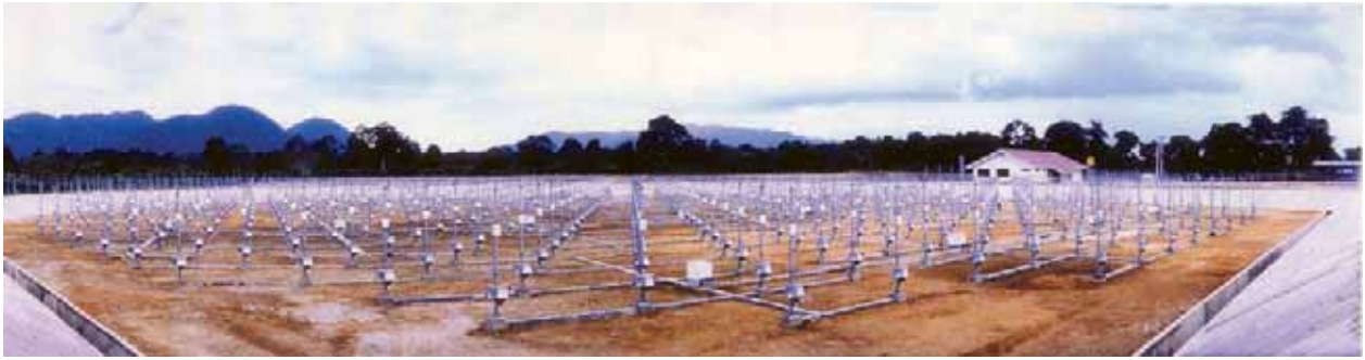
Figure 2. A view of the entire EAR.
